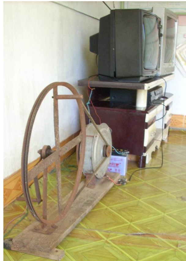
Figure 2. Audiovisual appliances (2 televisions, one VCR, voltage inverter operated on a 12V/4Ah motorcycle battery). In front: hand-operated generator to provide electric power if no wind is available 86 .
